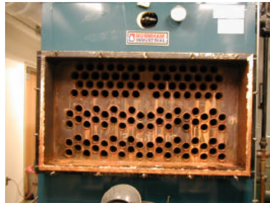
Condensation in a standard firetube boiler operating at 140°F on low fire.
