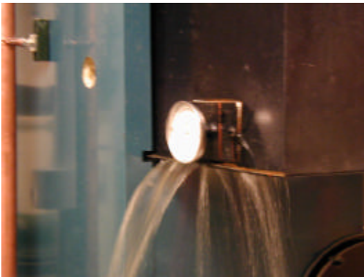
Condensation in a standard firetube boiler operating at 140°F on low fire.
