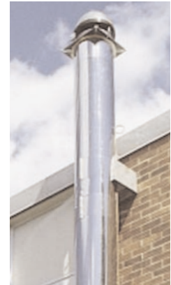
This installation is equipped with an end-of-the-line exhaust fan.
