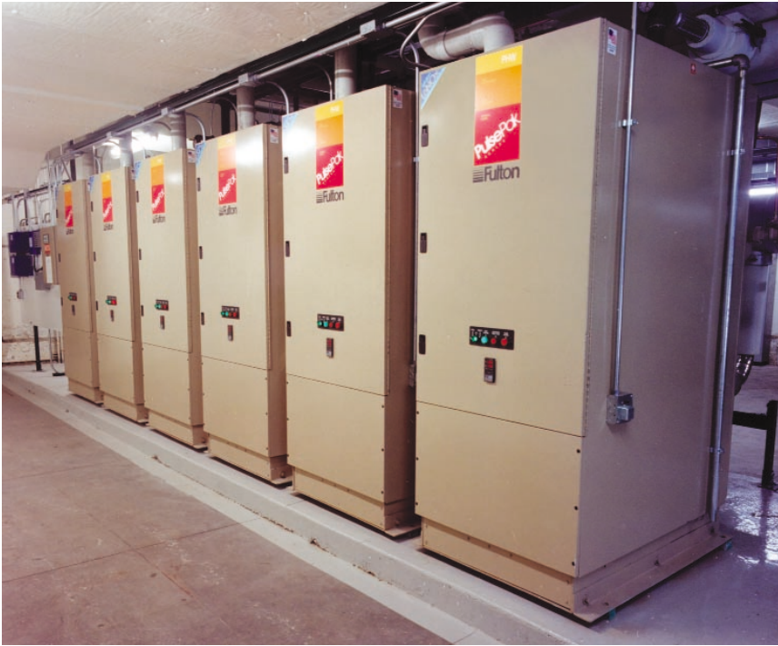
Shown above is a modular installation of six PHW1400 Fulton Pulse Combustion Boilers. Multiple boilers are staged to maximize the time spent at the lowest firing rate, thus maximizing efficiencies.
